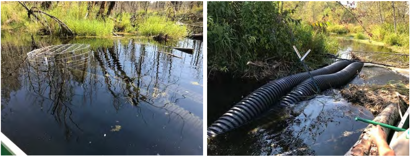
Figure 4. Examples of a flexible pond leveller with a double pipe configuration (images from Washington State Parks).
