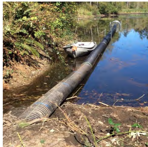
Pond Leveler Installation (Township of Langley, 2020)
