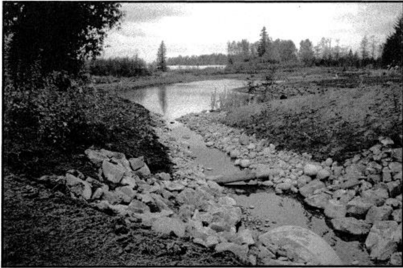
Photograph 5. Looking north at realigned channel south of constructed pond (October 13, 2000). Note riparian planting and hydroseeding.
